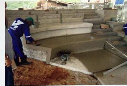
Mock up do Piso Floor Mock up, 04.2012
