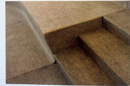
Mock up do Piso Floor Mock up, 04.2012
